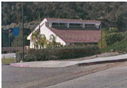
County of Riverside Fire Station #85 29405 Grand Ave. Lake Elsinore, CA 92530 951-245-2185
